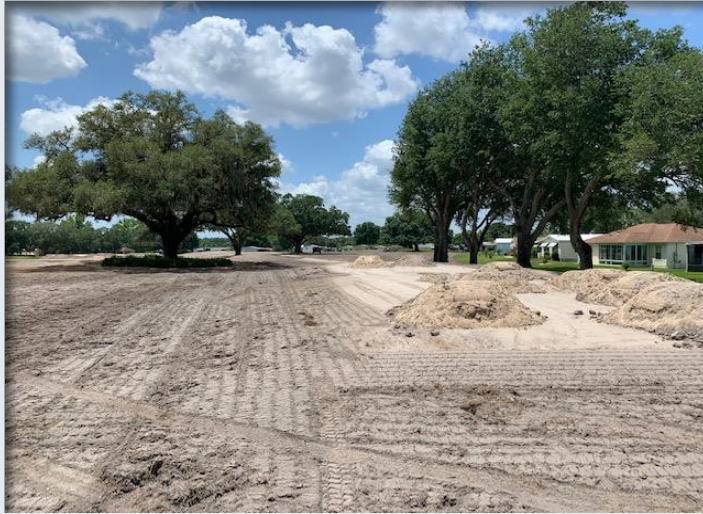
Adding soil material to adjust tee at #9
